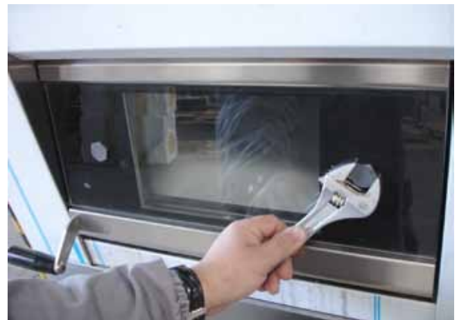
Fig. 3 Loosen the screws to substitute glass.
