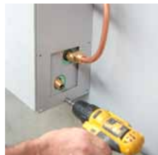
Fig. 6.2 Loosen the back panel.
