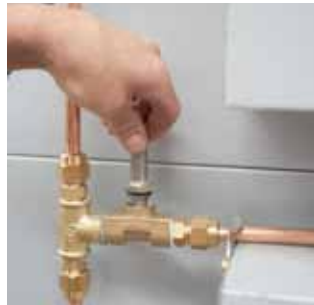
Fig. 7.4 Carefully remove the piston.
