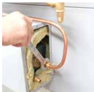
Fig. 6.3 Loosen the water input tube.
