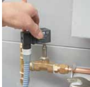
Fig. 7.2 Remove the coil.
