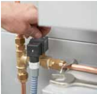
Fig. 7.3 Loosen the nut against the solenoid.
