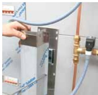
Fig. 6.1 Loosen the back steam output.
