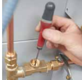
Fig. 7.5 Check if the piston is damaged or dirty, clean or substitute it. Reassemble the solenoid and open the water valve.
